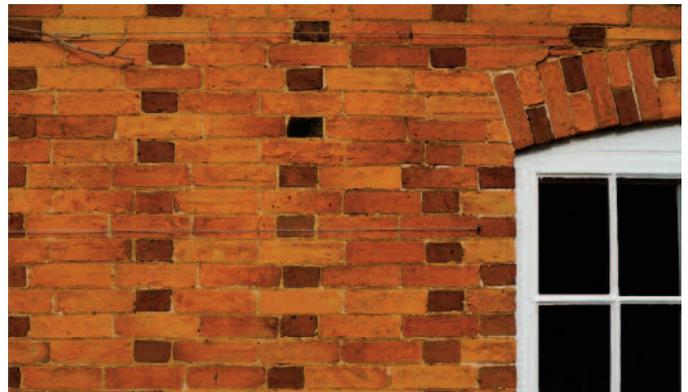
*Fig 34 Chequer brickwork*
