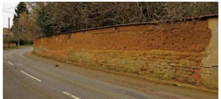
*Fig 38 Cob wall with capping on Teeton Road*
