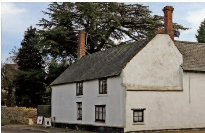
*Fig 35 Rendered cob cottage with rounded chimneys*
