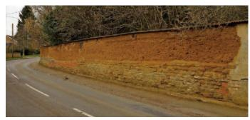
Fig 38 Cob wall with capping on Teeton Road
