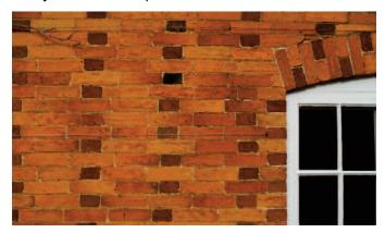
Fig 34 Chequer brickwork
